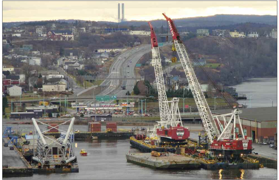
A floating dock at Pier 2 is used to outfit crane barges.
