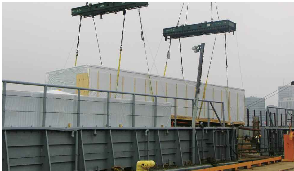
Well wrapped modular homes made in Fredericton are transported to Nunavut by barge.
