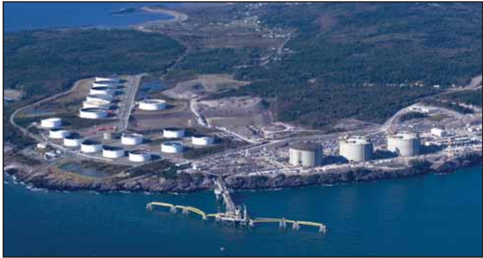
Canaport LNG is prepared to receive the first MOSS tanker at the jetty above in early 2009.
