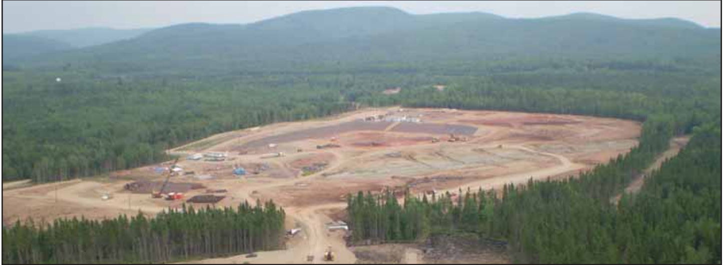
The Picadilly site, as viewed from the head frame building.
