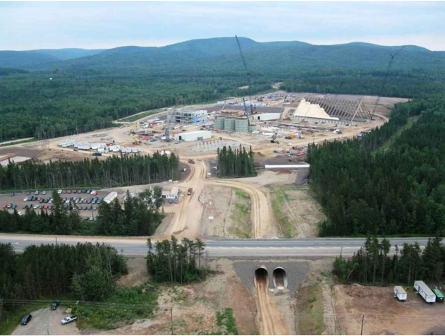
The Picadilly Potash mine construction is on target for production in 2010.
